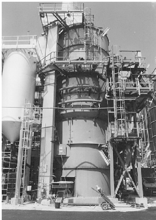
Fig. 3. FBC plant during installation.
